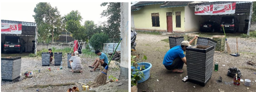
Gambar 8. Proses Pengecatan Bak Sampah
