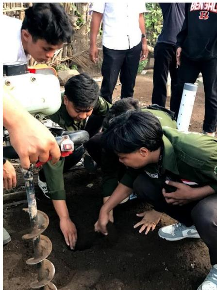
Gambar 3. Penanaman Lubang Resapan Biopori
