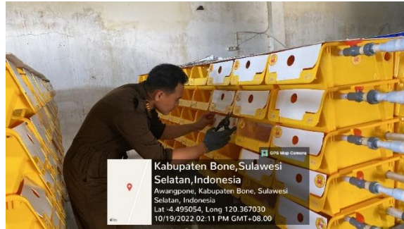
Figure 2. Maintenance door installation
