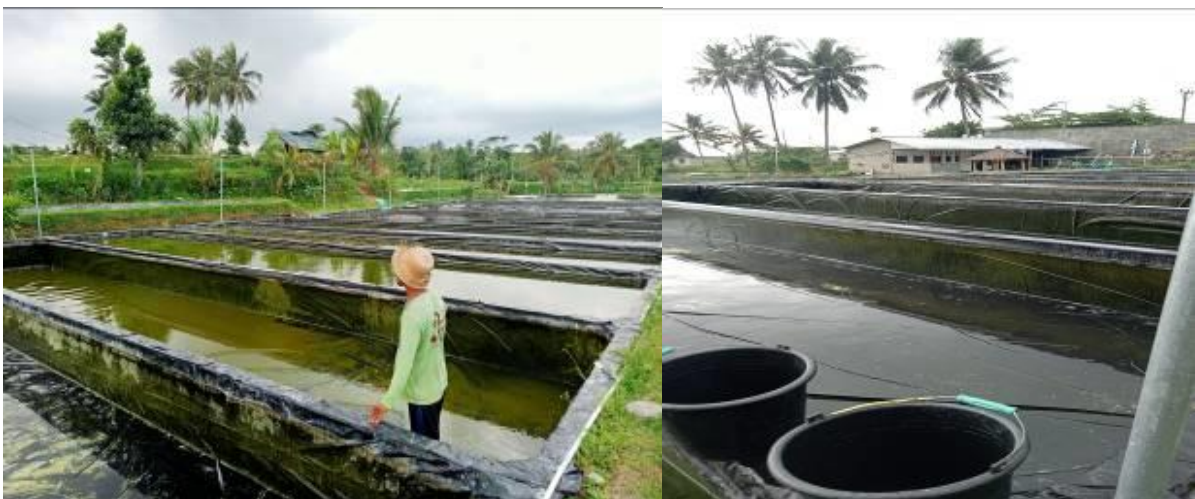
Figure 2. Pool draining and cleaning
