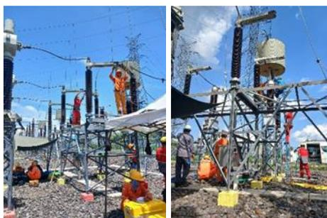
**Gambar 1.** Kegiatan Pemeliharaan *Shutdown Measurement* Bay Line Sengkol 2 GI 150 KV Kuta
